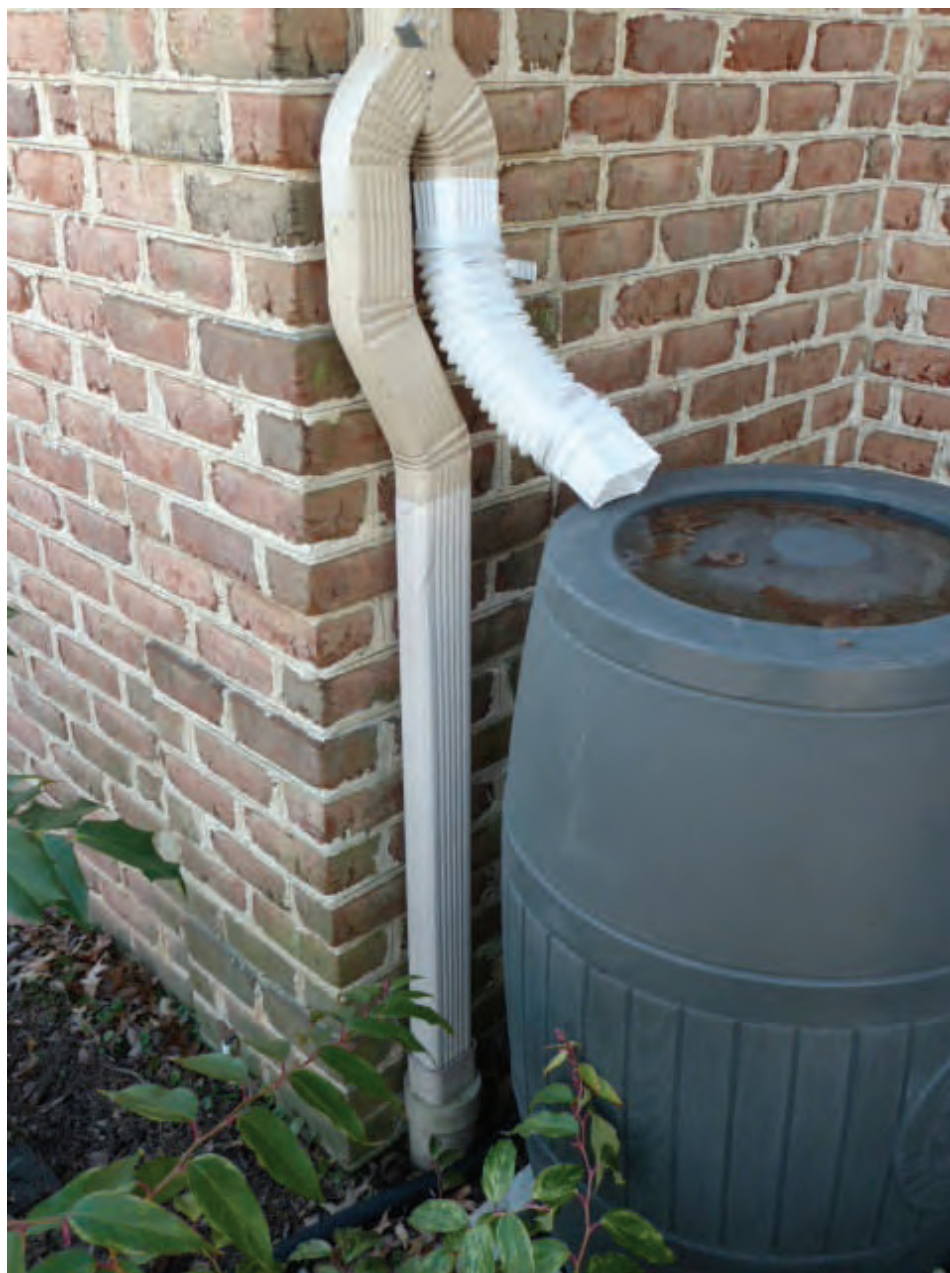
Rain barrel diverter and flexible downspout tubing are used to direct rainwater into the rain barrel in season for capture and use in the garden.
