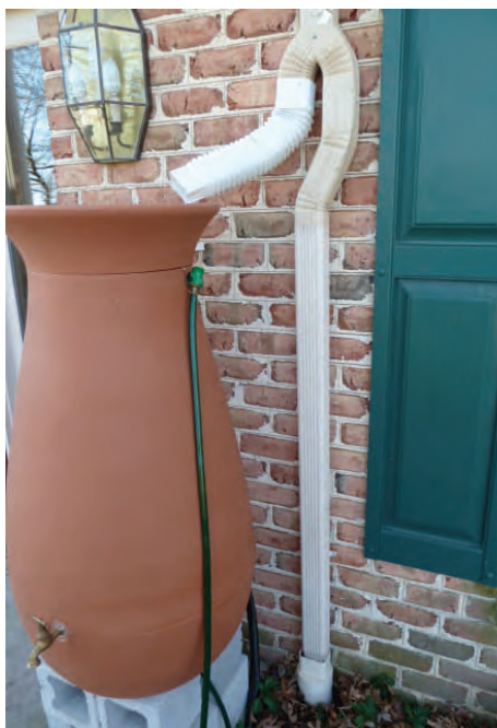
Rain barrel diverter and flexible downspout tubing.
