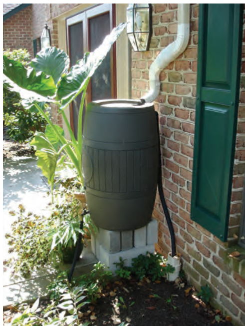
Rain barrel installation using a flexible tubing downspout.
